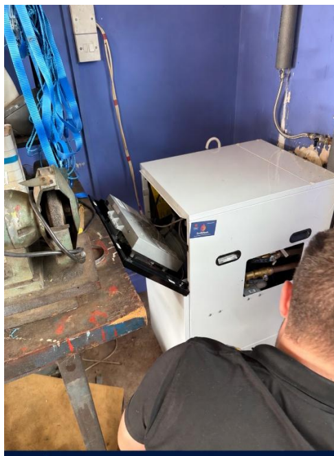
2 Engineer carrying out the repairs
